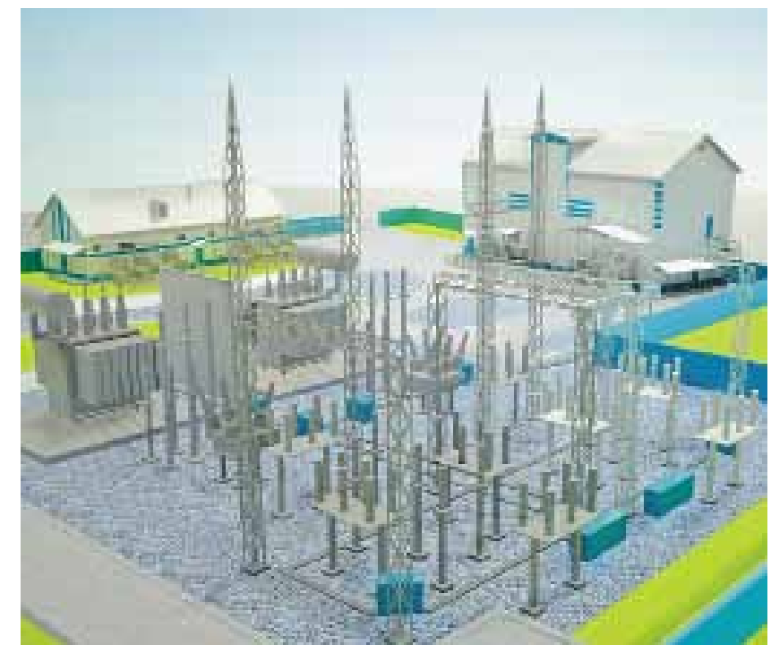
110/10/6 kV "Zapadnaya" conversion and distribution substation
