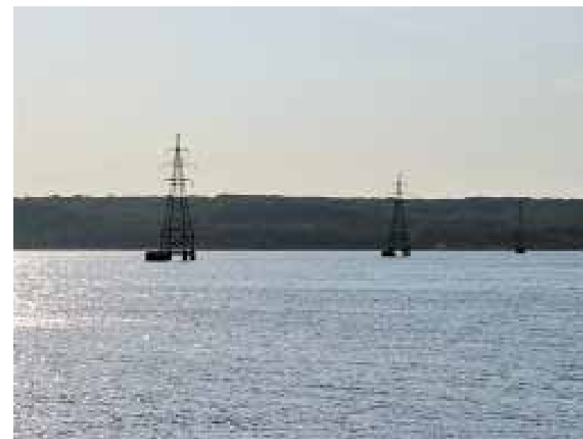
110 kV overhead transmission lines No. 9,10 (crossing over water reservoir)
